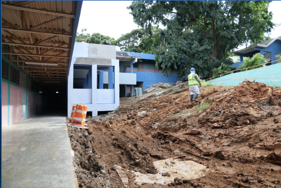
José N. Gándara School, Aibonito $2.6 M
