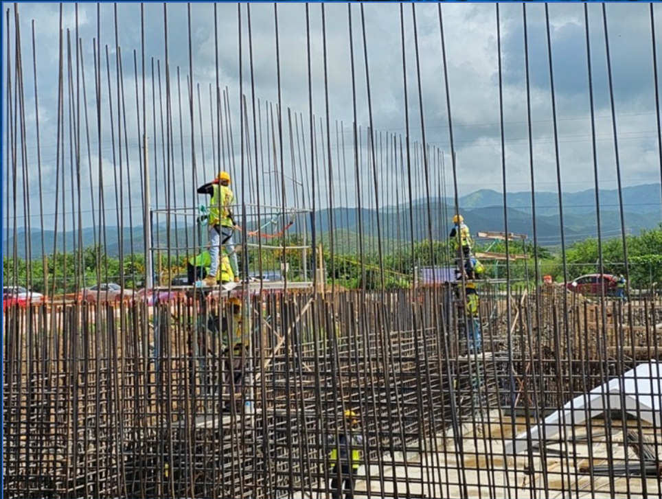
Regional Sanitary Plant, Guayama $93 M
