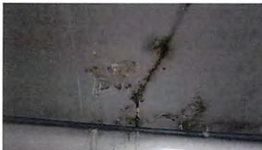
Figure K2: More previously installed failed injection repairs with leaching forming
