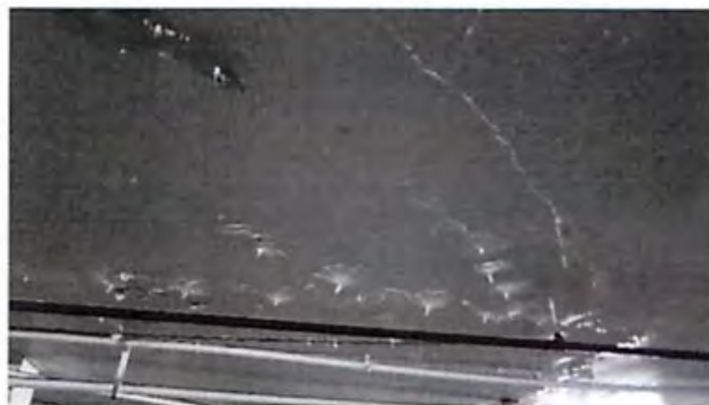
Figure K1: Previously installed failed injection repairs with leaching forming
