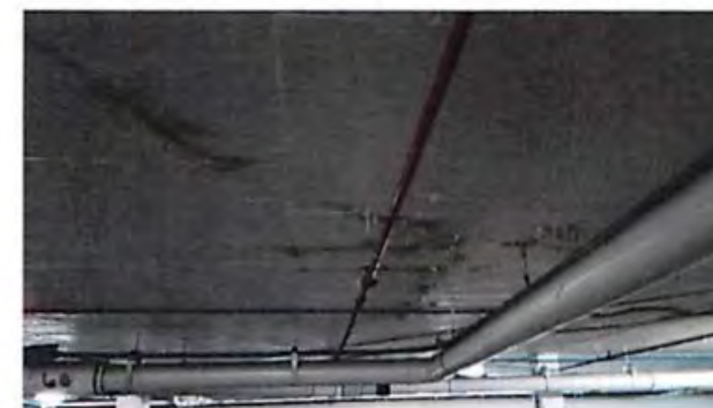
Figure K2: More previously installed failed injection repairs with leaching forming
