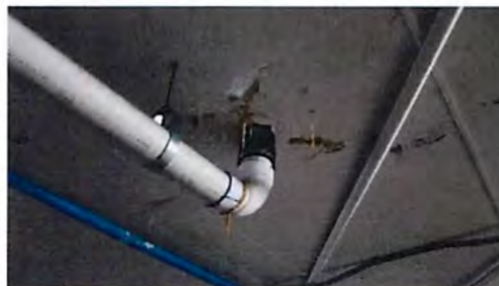
Figure K1: Previously installed failed injection repairs with leaching forming
