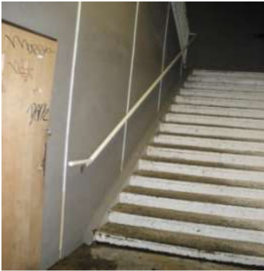
Parking Exit Stairs
